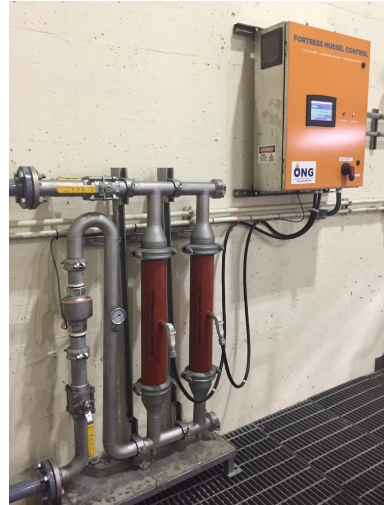
20 MGD copper ion generator installed in Lawrence, KS
