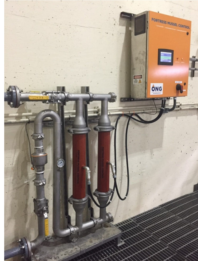
20 MGD copper ion generator installed in Lawrence, KS
